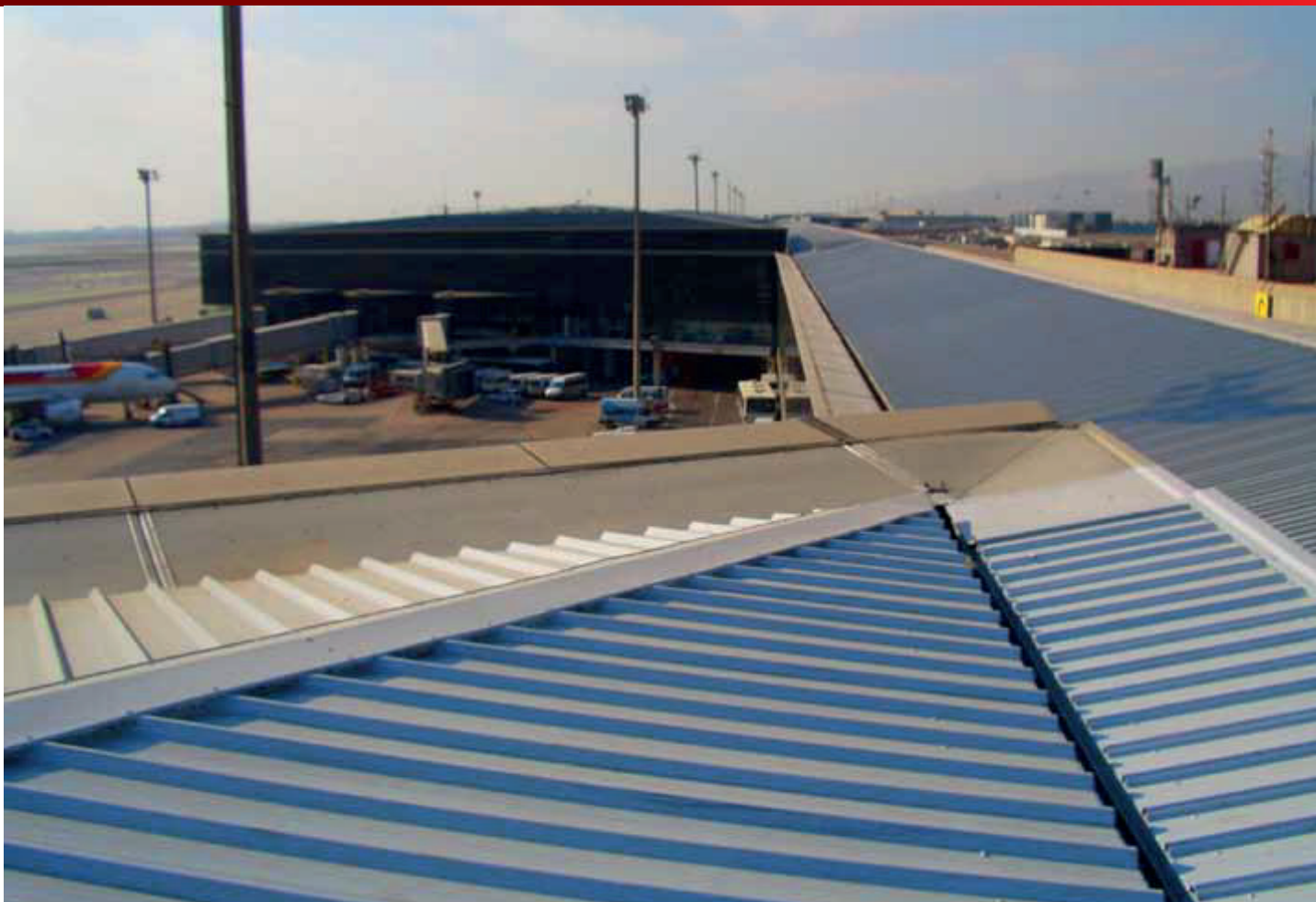
BARCELONA AIRPORT ROOF, SPAIN, 18,500 M 2 .
