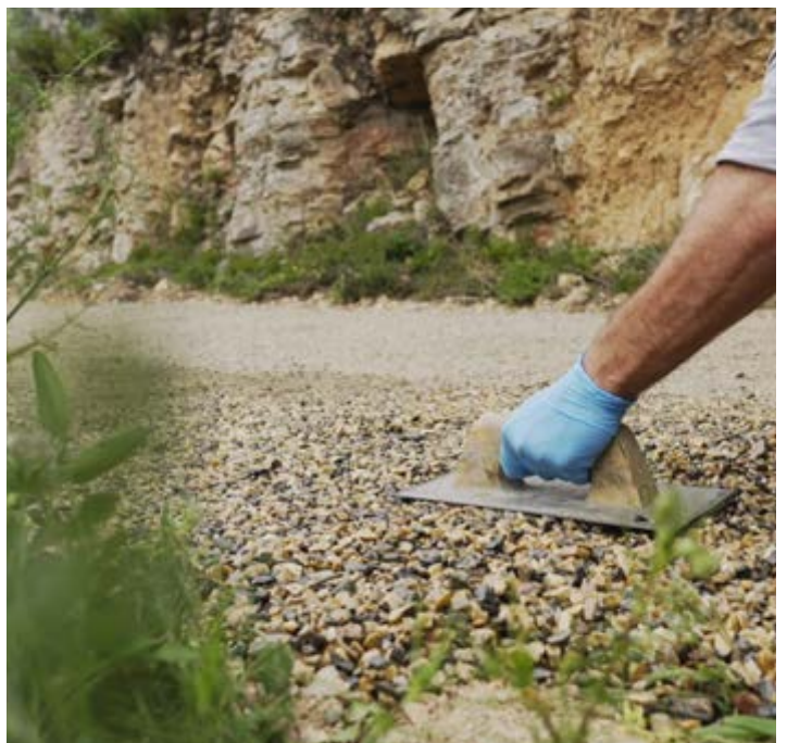
FLOORING ON A PERI-URBAN ROAD, VANDELLÒS, SPAIN
