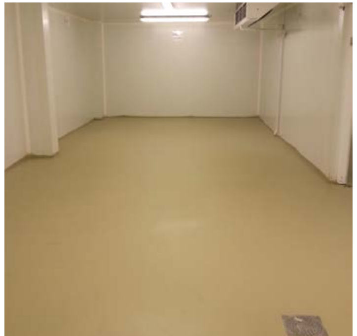
REFRIGERATED PROCESS ROOM, FRANCE, 1.400 M 2
