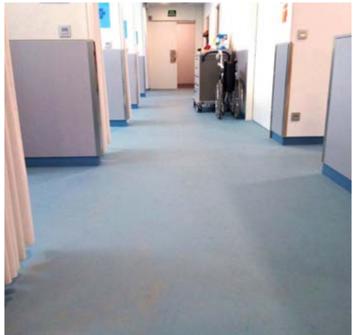
HOSPITAL AREA FLOORING, ANDORRA, 400 M 2
