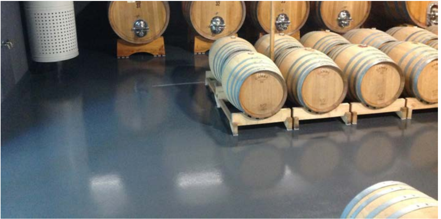
WAREHOUSE FLOORING, ITALY, 300 M 2
