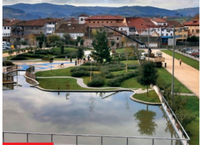
Rainwater drainage pond waterproofing in the Pelambre Park. Villaviciosa, Asturias, Spain.
