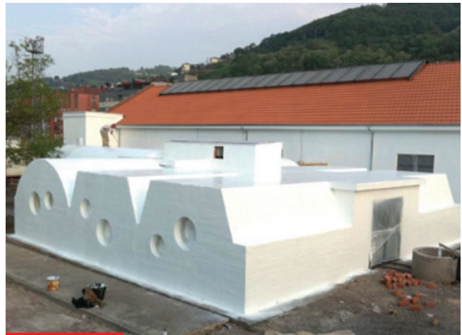
Simulation tunnel at the Miners' Training Centre, Oviedo. Spain
