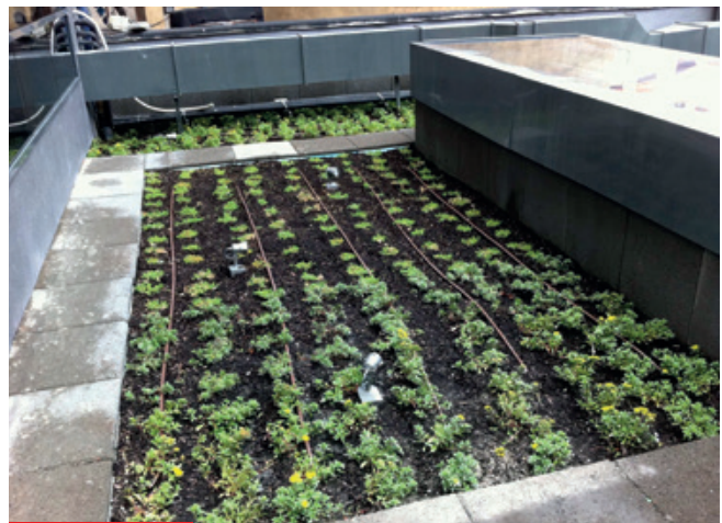
Green roof on the Regional Health Ministry building, Oviedo. Spain.
