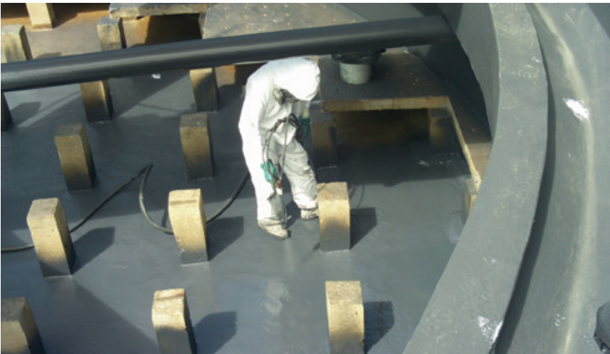
Polyurea waterproofing membrane application on a wastewater treatment tank.
