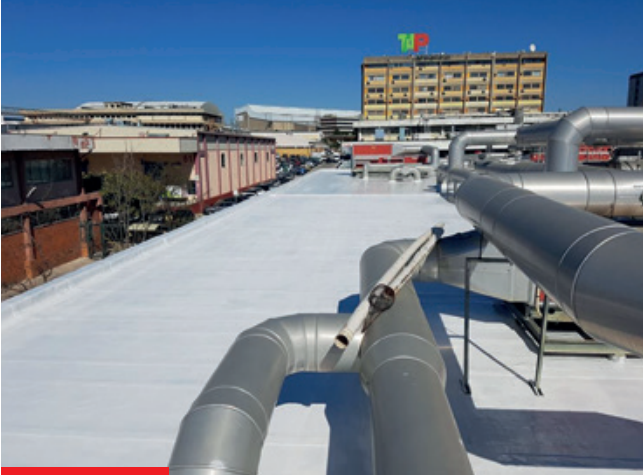
Lisbon Airport building roof waterproofing. Portugal
