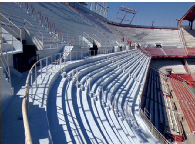
Football Club Sevilla Stadium stands waterproofing, Sevilla. Spain.
