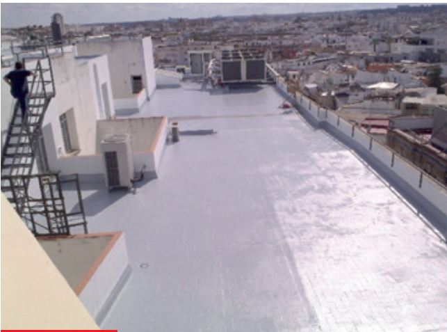
Residential building roof waterproofing in Andalusia. Spain.
