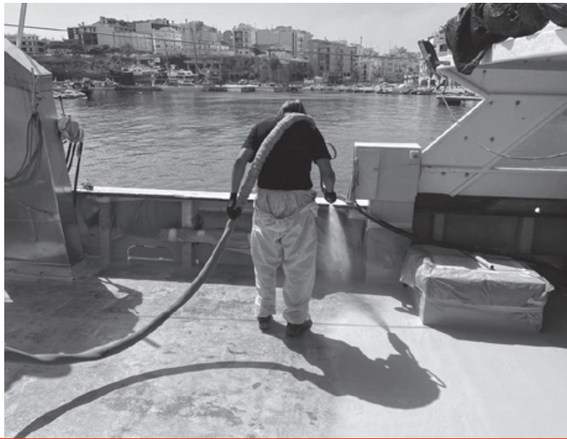
Corrosion protection with polyurea on a boat deck.
