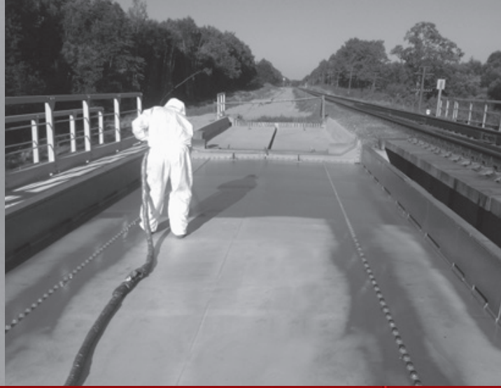
Waterproofing of a bridge deck in Latvia.
