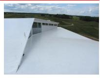
waterproofing membrane (without joints or overlaps), of high mechanical and external resistance, thermoset and elastomer (with the ability to bridge the possible fissures of the support). The coating, once cured, is inert, free of hazardous materials and heavy metals, making it fully recyclable at the end of its useful life. The membrane heals in a few seconds and its commissioning is
